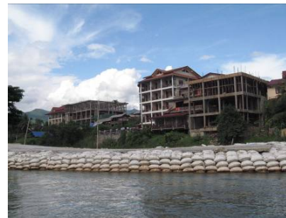
Multi-storey hotels under construction
