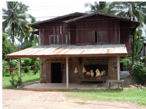
Two storey dwelling; stone and timber finish
