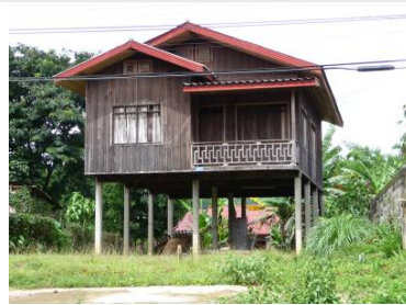
Elevated single storey dwelling; timber finish
