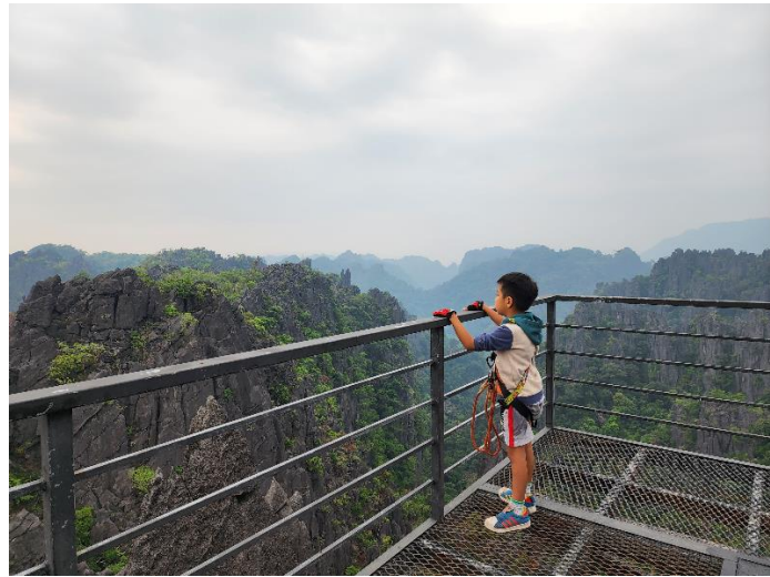
The Rock Viewpoint, Laos: Steel viewing platform and small swing bridges provide safe walking and viewing opportunities on steep limestone, similar to that found in Vang Vieng. Although these structures at The Rock are associated with a guided zipline tour, similar structures could be installed at the viewpoints in Vang Vieng to make access easier and walking along ridgetops safer.
