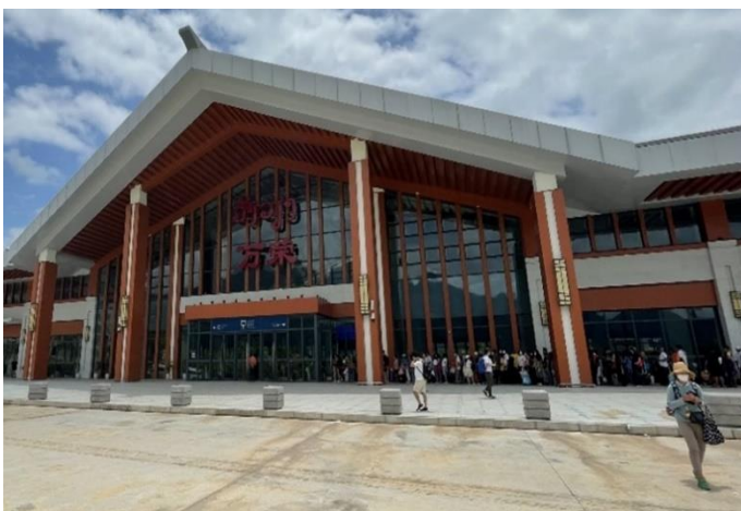
View of new Railway Station
